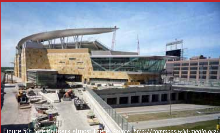
Figure 50: Site Ballpark almost there Source: http://commons.wiki-media.org/
