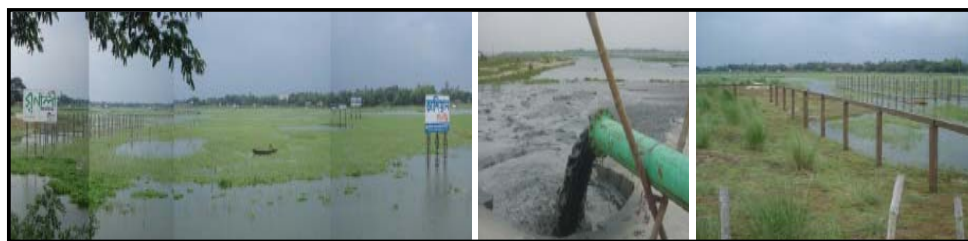
Land filling and ongoing development by encroaching wetlands
