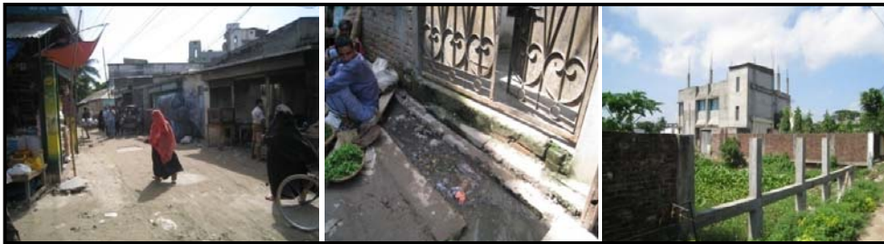
L-R: No drainage system in secondary road, clogged drain, encroachment of wetland.
