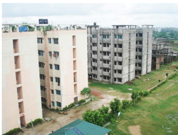
Entrance of the project
