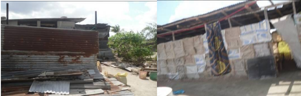
Figure 8 Temporary houses while occupants await the completion of the main building
