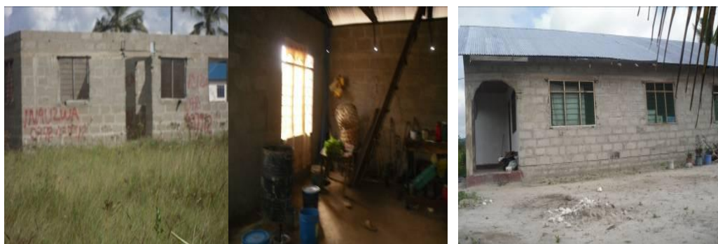
Figure 7 Unfinished buildings due to inadequate money
