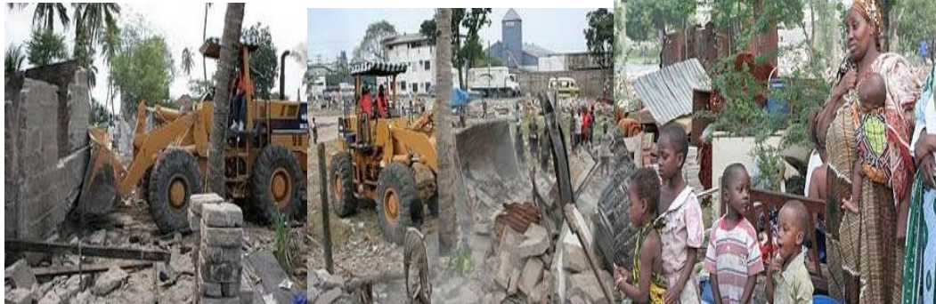
Figure 12 Demolition of buildings and properties at Kipawa
