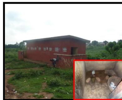
Figure 5: KVIP toilet Block at Affordable Housing Project
