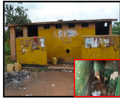
Figure 4: Ordinary Pit latrine at Zicco toilets
