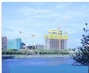
Construction on the Ostend
