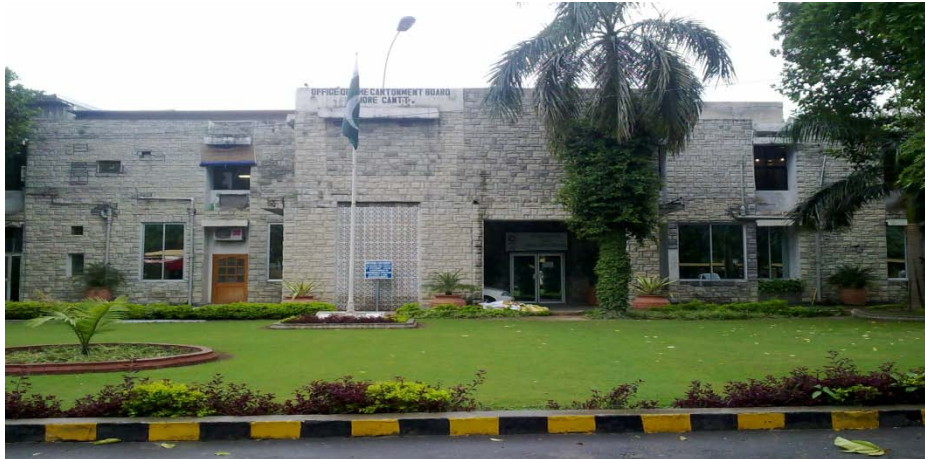
The main office block of the LCB
