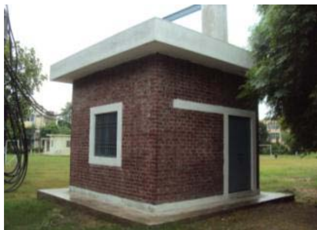
Tube well Room
