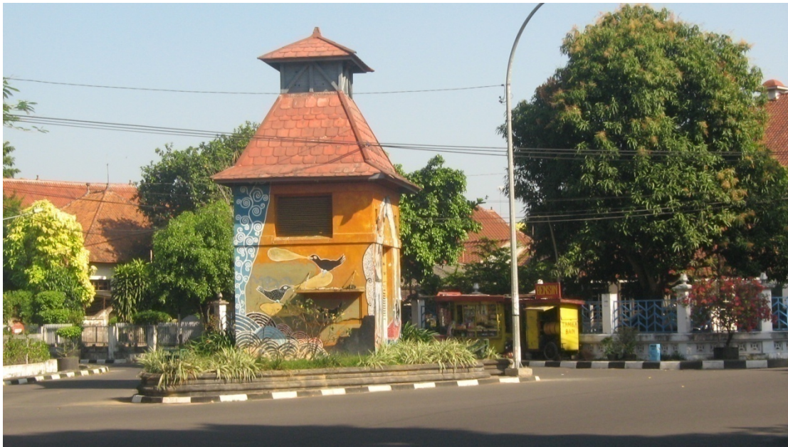
Figure 3.5. Mural on the Walls of an Old Powerhouse
