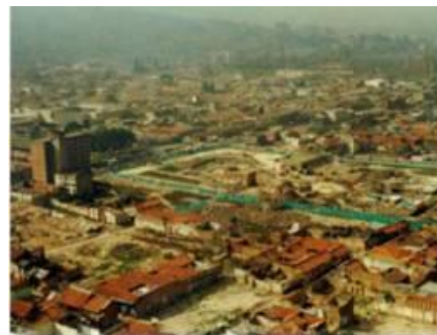
Figure 8: View of the Santa Inés neighborhood and El Cartucho sector in Bogotá D.C. during the construction of the Third Millennium Park
