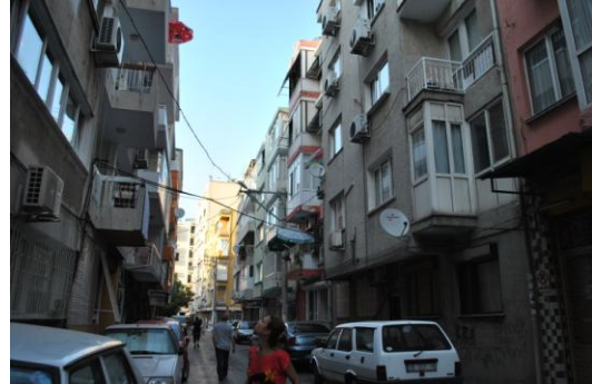
Fig.4. 13: Air-conditioners on facades
