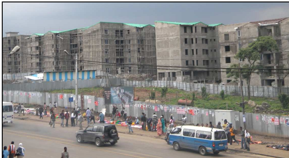
Figure 4.2 The Low Cost Condominiums Built on the Site (After the Project)
