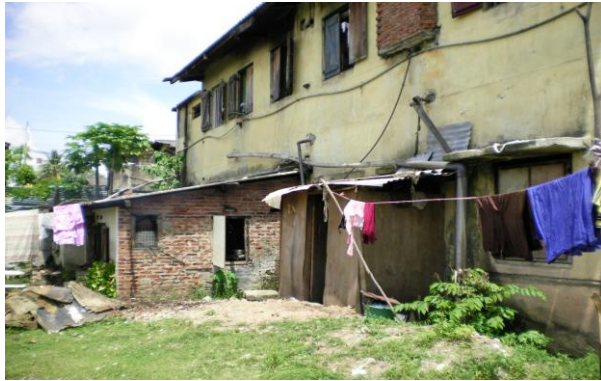
Figure 22: Un-authorized additions to low cost flats
