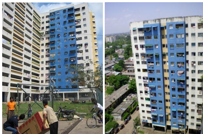
Figure 8: External view of the “Sahaspura” condominium building
