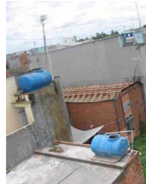
Picture 3-15: Water tanks on the top of houses found in C.U.120
