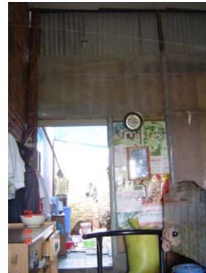
Picture 3-7: Temporary materials used in a house in C.U.16
