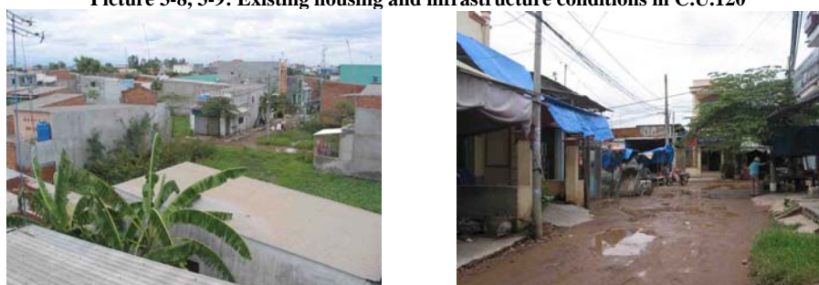
Picture 3-8, 3-9: Existing housing and infrastructure conditions in C.U.120
