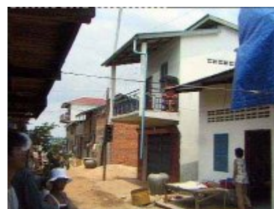
Figure 22. Phnom Penh 1997-99: Voluntary demolition → Planning → Relocation of roadside shacks. Photo from ACHR website
