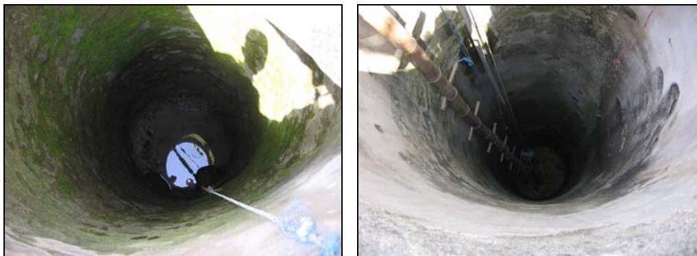
Figure 5.9. The Condition of groundwater wells after the sumur resapan construction
