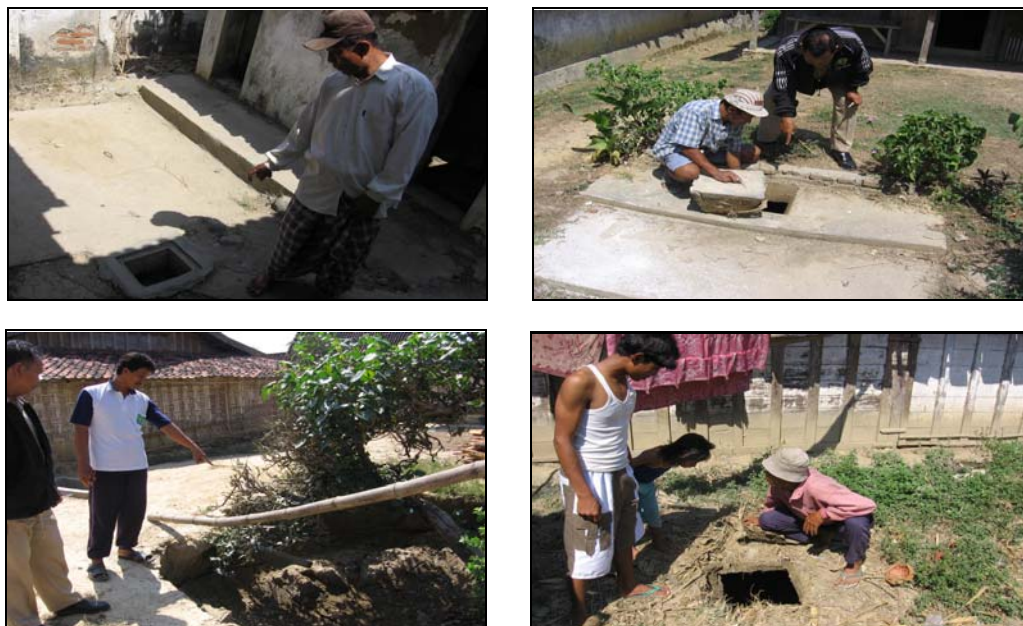
Figure 5.2. Existing Condition of the Sumur Resapan in Kragan District
