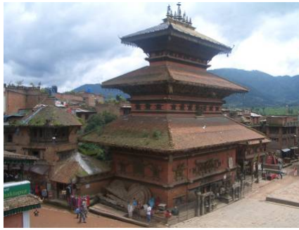
Figure 9: Dattatraya Temple which was devastated in earthquakes because of low plinth (picture taken from the top plinth of Nyatapola in Bhaktapur)
