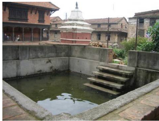
Figure 16: Pokhari the water reservoir in community space in Harisiddhi, Lalitpur
