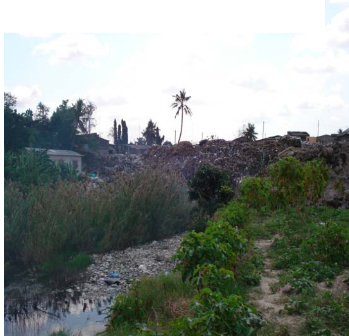
Image 1: Leachate flow to Msimbazi river valley At Kigogo dumpsite
