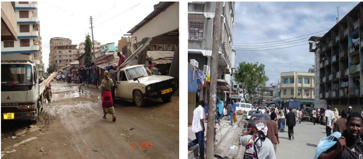
Photograph 5: Deteriorating and un-maintained infrastructures
