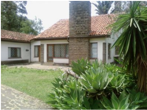
Figure 4-3: Typical single family unit
