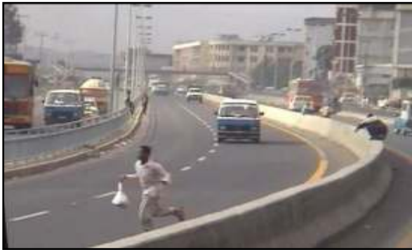
Figure 4-17: Accessibility problem occurred as a result of the Ring road construction
