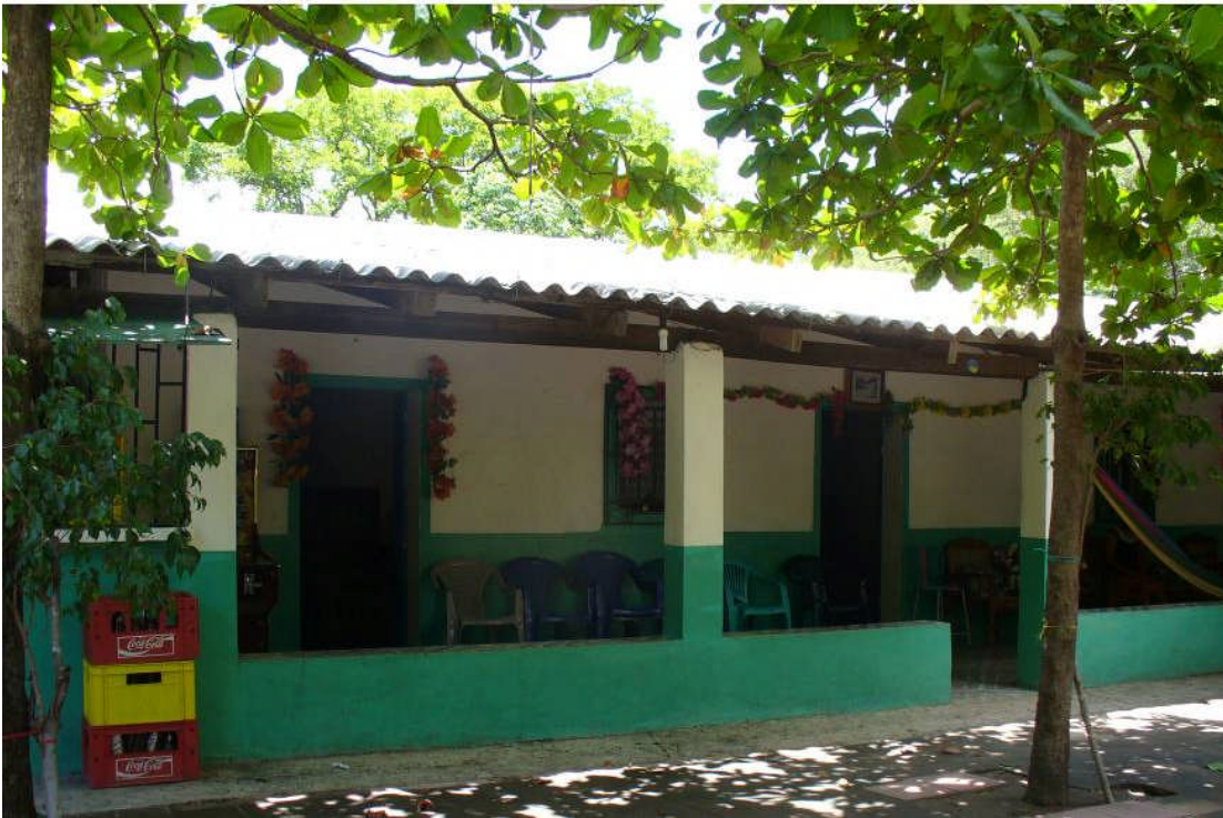
Comparison of unrenovated and renovated houses of a similar type on the same street. Both are adobe construction, but the house below has stuccoed, painted, and replaced the roof, floor, windows, and doors.
