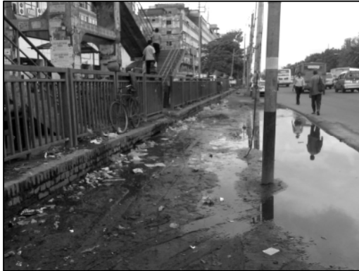
Figure 6.18: The inefficient drainage management
