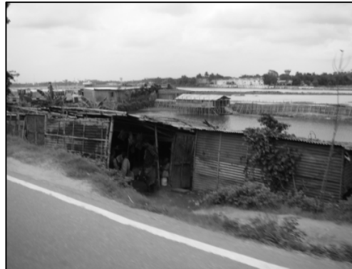
Figure 6.15: illegal structures on the western embankment
