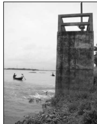
Figure 6.17: The Sluice gate near Goran Chatbari pump station
