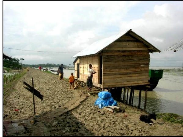
Figure 4.3: New construction again outside dam (notice the river in the background), Southkhali Source: Author
