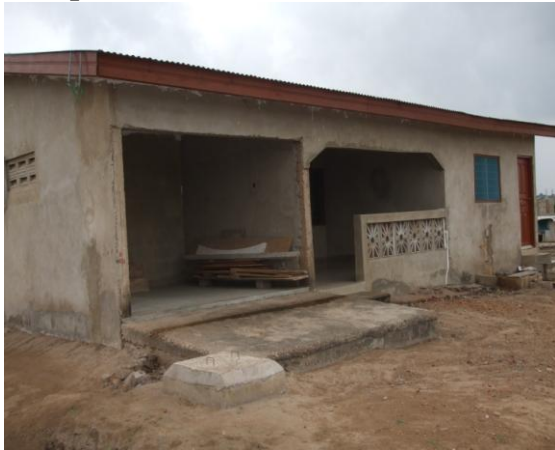
Image 1: floor tiles Completed house
