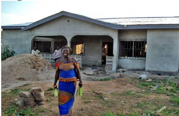
Image 2: House under construction
