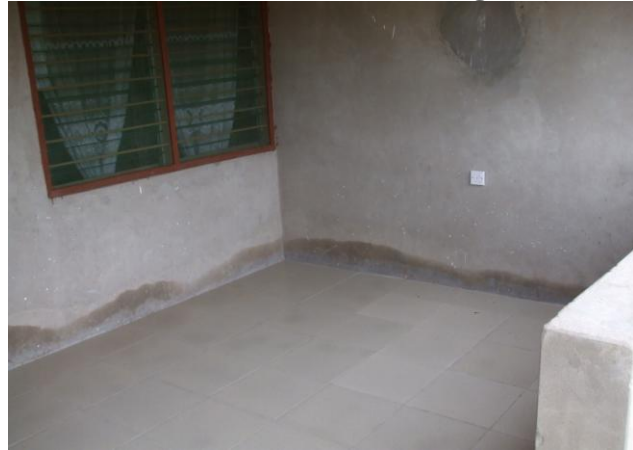
floor tiles fixed after roofing
