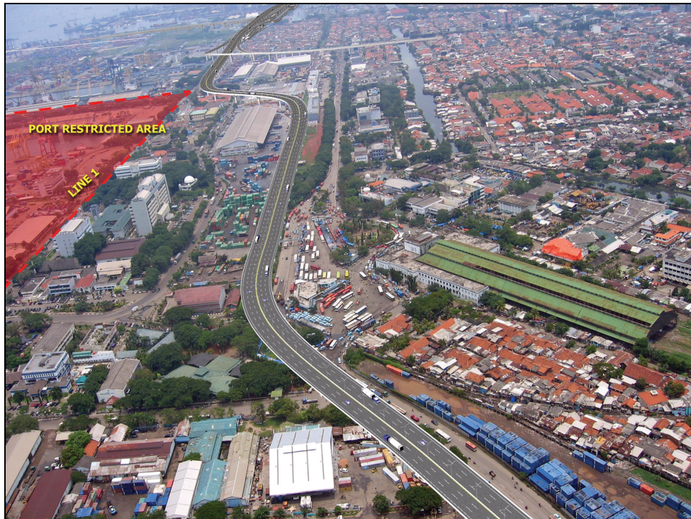
Figure 39. Tanjung Priok Access W-1 and W-2 Sections (Source: Ministry of Public Works, 2009)
