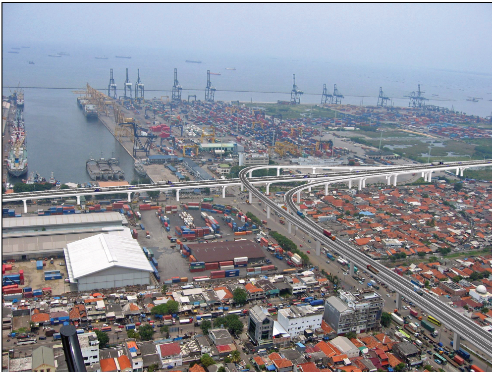
Figure 38. Tanjung Priok Access E-2, W-1 and NS Sections (Source: Ministry of Public Works, 2009)
