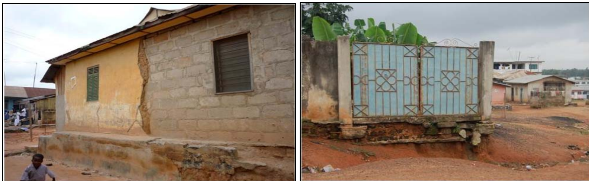
Left Photo: House with original structure made of mud at the left and new structure made of sandcrete at the right half; Right Photo: Foundations of a fence exposed already because of erosion.
