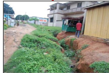
One of the roads with drainage gullies
