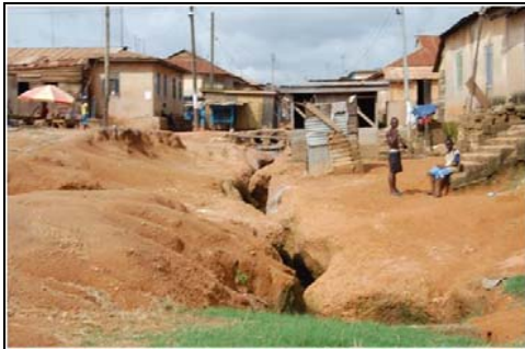
Deep gully drainage going to the direction of the river on the west of Ayigya.
