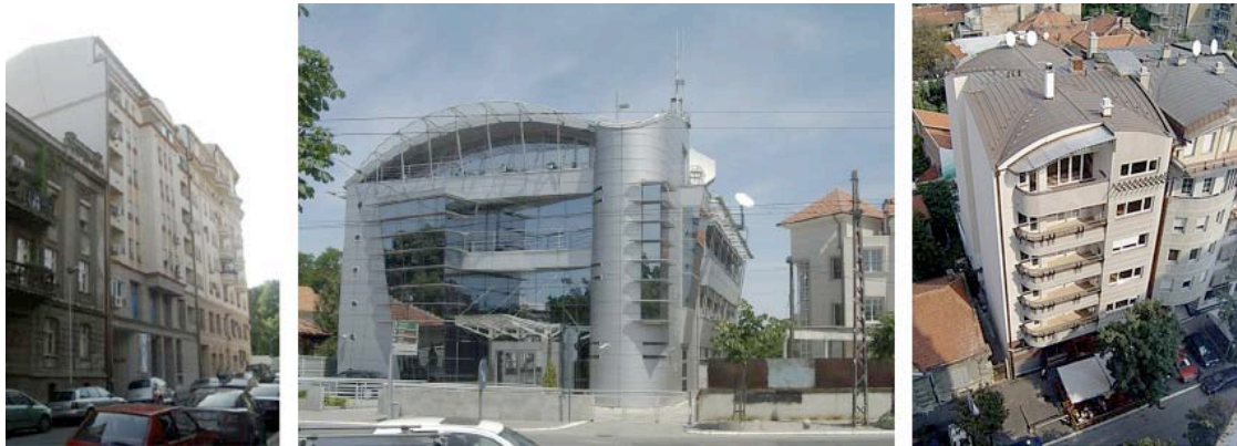
Figure 18: Exceeding the allowed size of the object – in the densely populated areas in the city centre (left), commercial (centre) and hi-rise residential (right) buildings in the low-density residential areas
