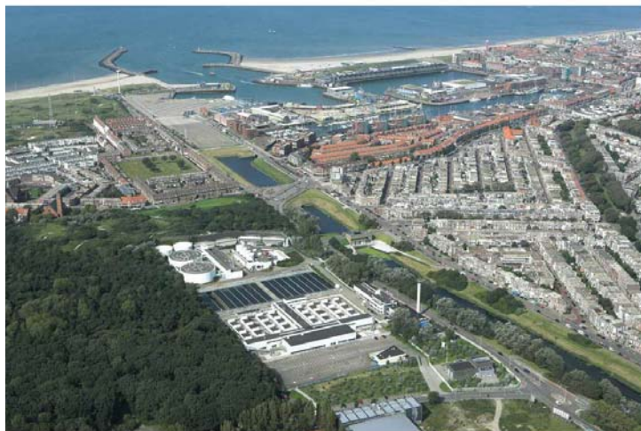
▲ Figure 44 Aerial Photo of Houtrust Plant Source: Aeroview Rotterdam
