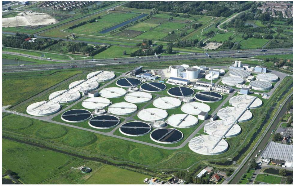
▲ Figure 44 Aerial Photo of Harnaschpolder Plant Source: Aeroview Rotterdam
