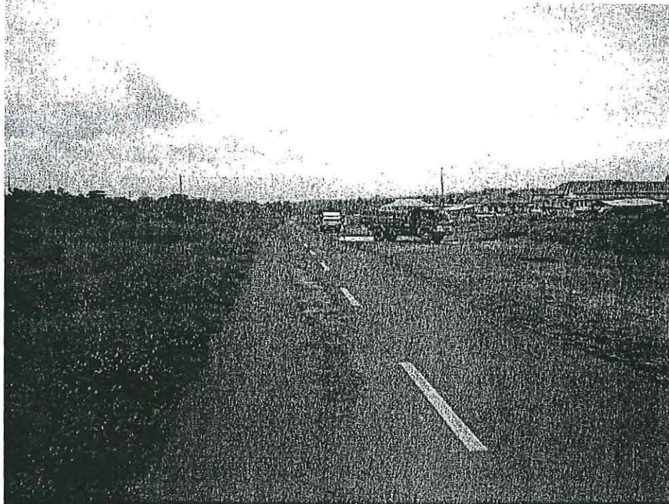
Figure 9 Main road project in Saumlaki town
