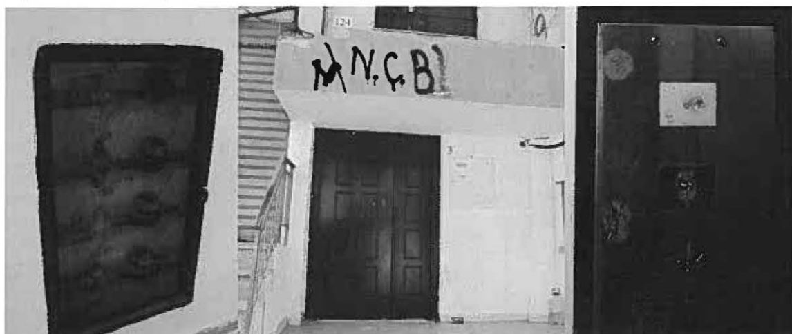
Figure 11: Common problems in newer buildings
