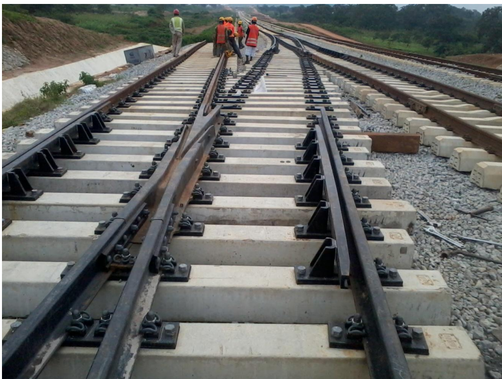
Annex 5: Photograph showing Rail track at Ring Road Two
