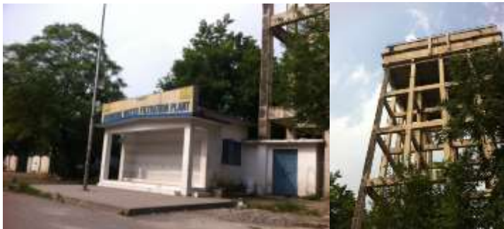
Photograph 15: Water filtration plants and overhead water tanks for the area
