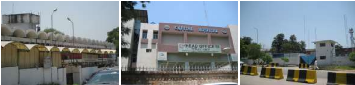
Photograph 14: Public facilities G-6
