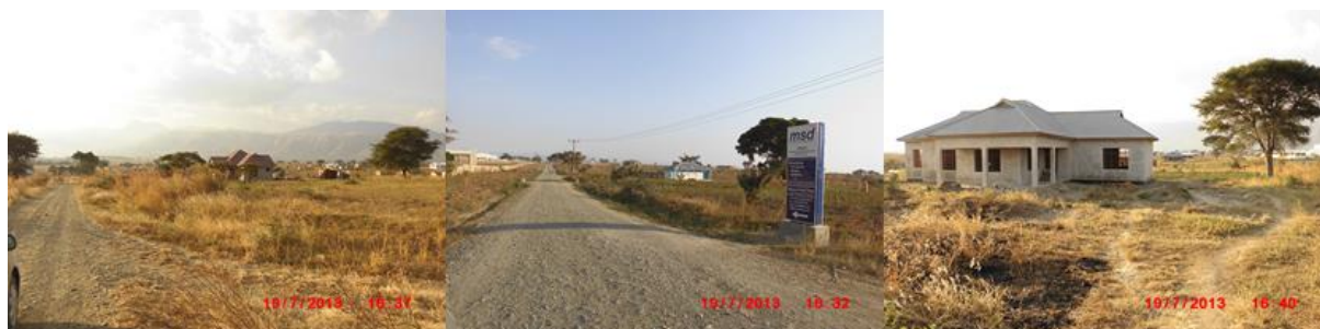
Figure 12: Pictures showing some parts of Iwambi area with an on-going construction of houses
