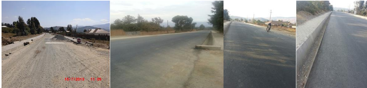
Figure 14: Picture of the road during and after road construction
