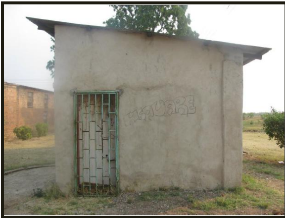
Renovated Toilet at Chikalabwamba Market in Mufulira
