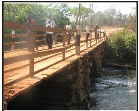
ACP Bridge constructed in Solwezi
