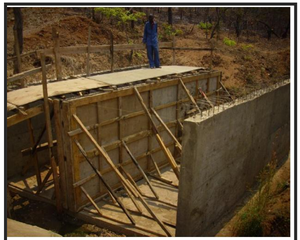
Bridge under construction in Mponda
