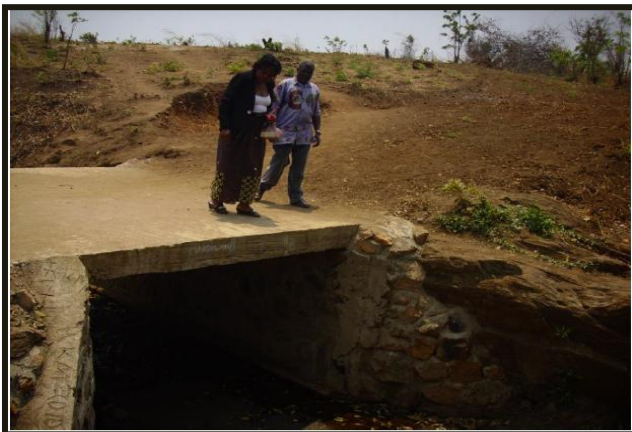
Bridge constructed at Mponda in Katete.
