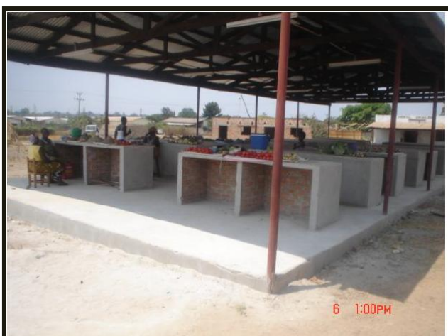
Market Shelter constructed in Luanshya (Source: CARITAS Zambia, 2011)
