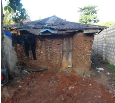
Figure 8: Mud-walled artisanal fisherman's house. Note adjacent concrete wall (to the right) indicating on-going (encroaching) development
