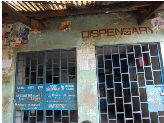
Picture 3: Upendo Dispensary
