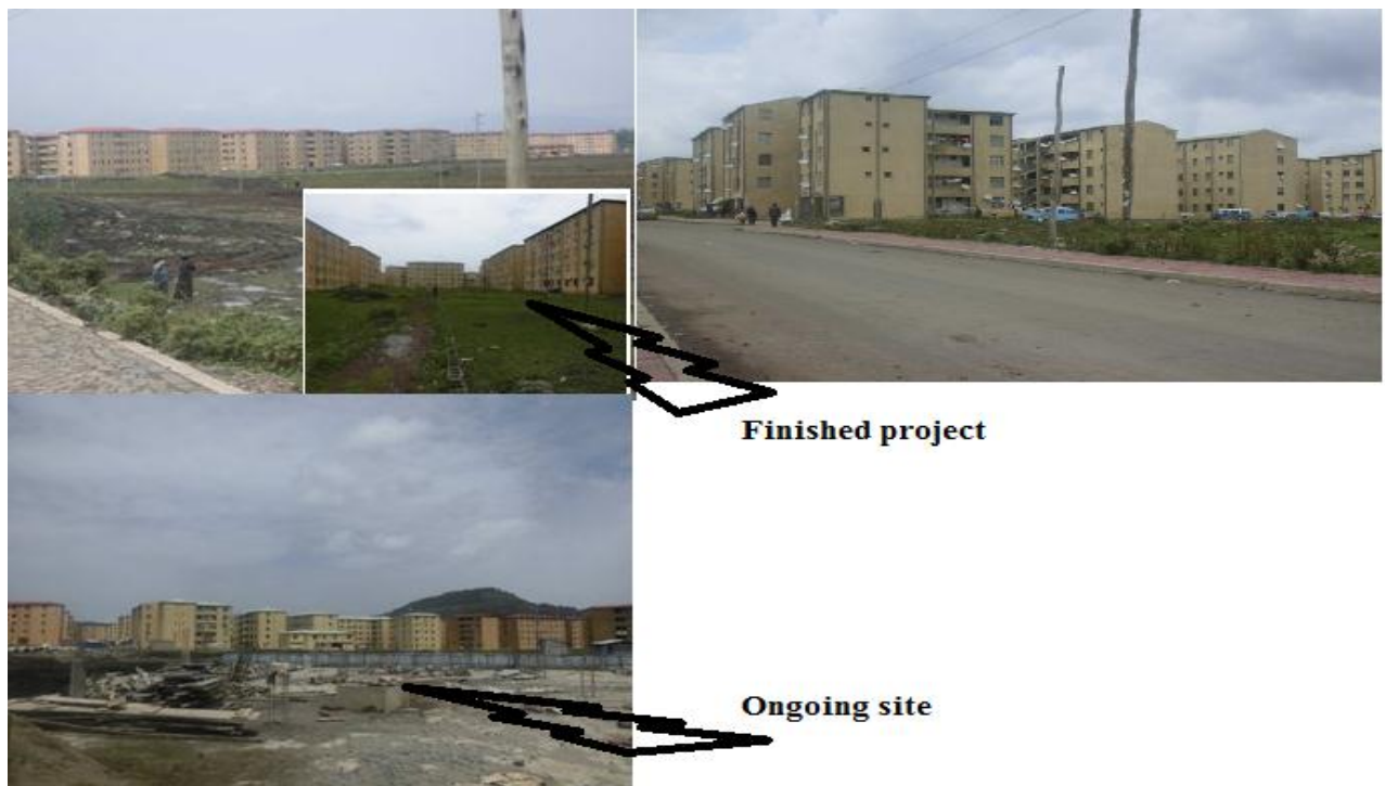
Figure 7: Gelan I and II project
