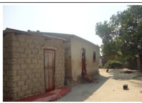
Figure 10: Typical Basic Mud Brick House
