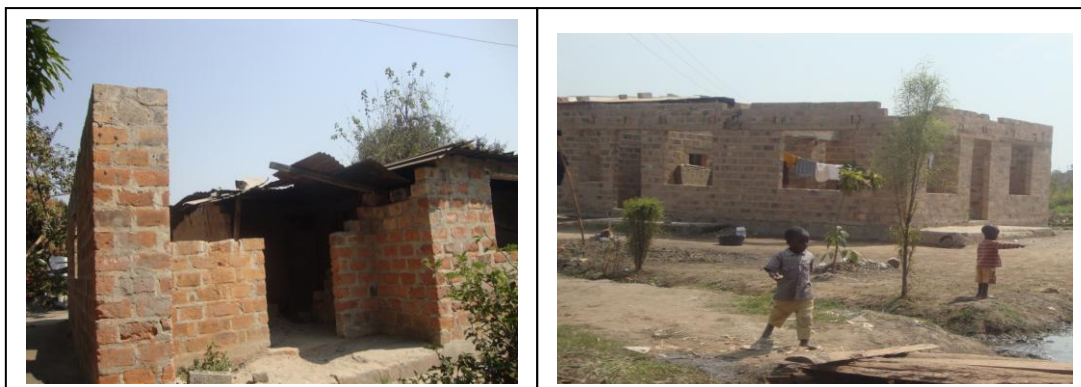
Figure 14: Typical Brick House under Construction as Family Lives Inside
