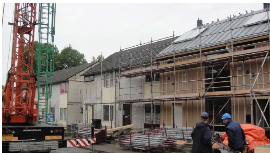
Renovation in progress
