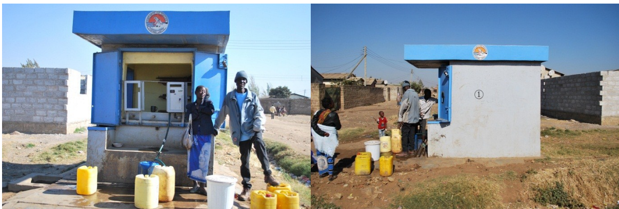
(b) Closed water kiosk
