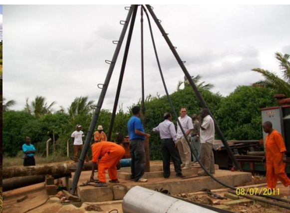
Figure 31 Hoisting of pumps in Tiwi wells , (Source; Mowassco Records, 2012)
