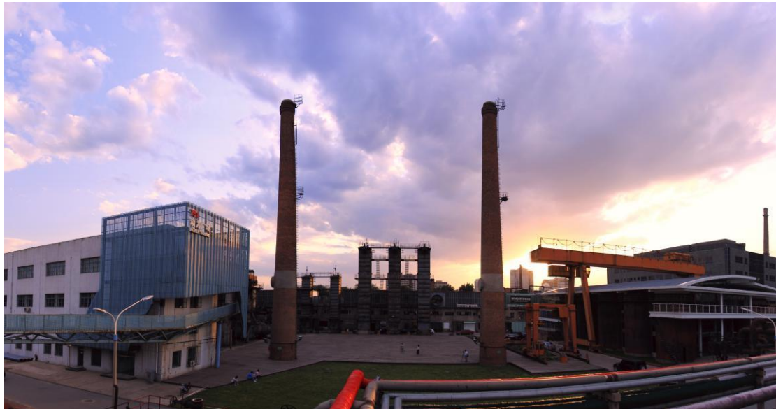
FIGURE 3: Power Square in 751 D Park
