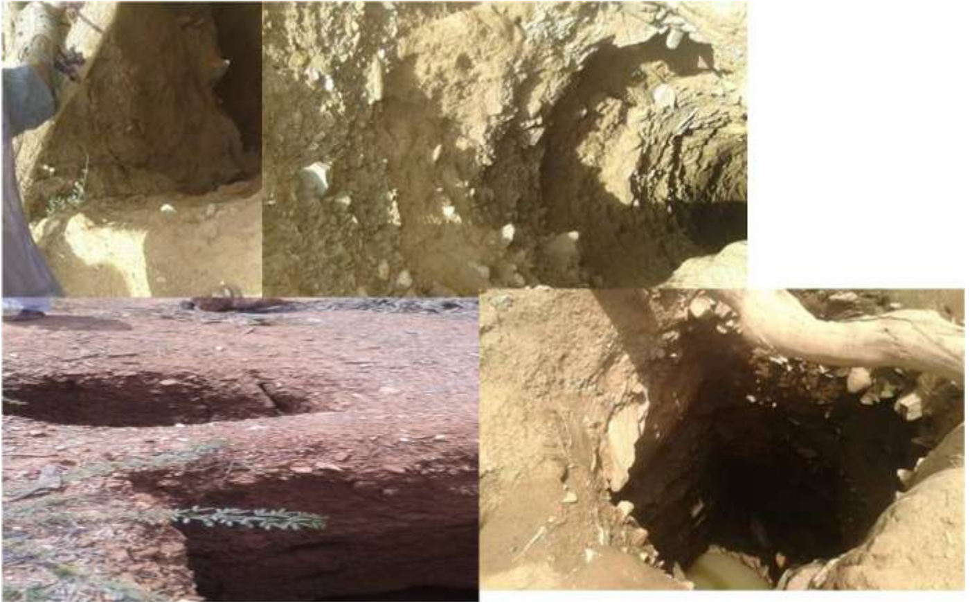
Figure 4 Risky Pits in Hademdemi Site
