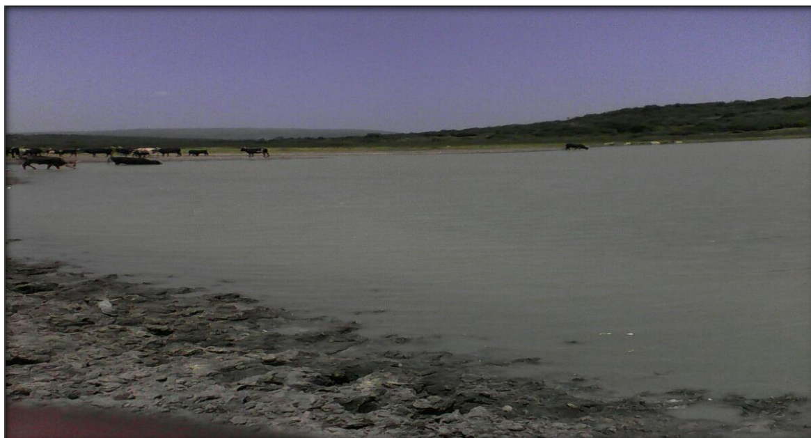
Picture 5: A dam constructed by government on a rangeland in Makukuru in Lyantonde
