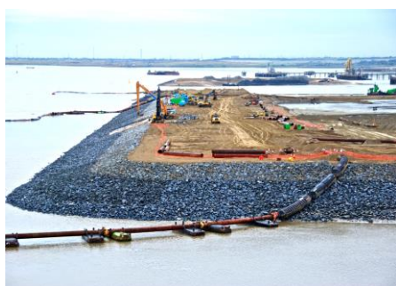
Figure 27 - Construction of slope protection in a port (source: The maritime Journal)
