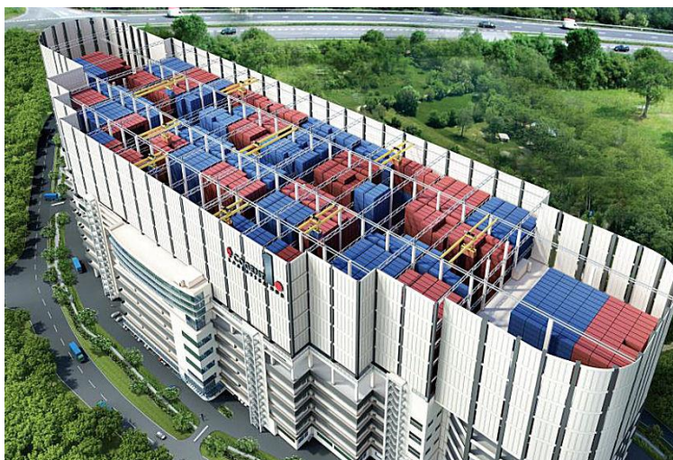
Figure 5 - One stop integrated logistic hub with warehouse, distribution and container depot on the rooftop (source: Jack-era.com)
