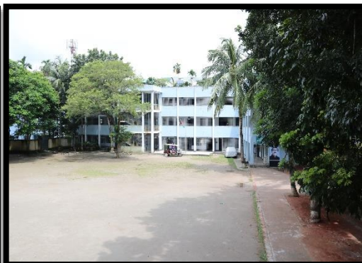
Photograph 5: Concrete built classroom at Govt. school (Photo credit: Author)
