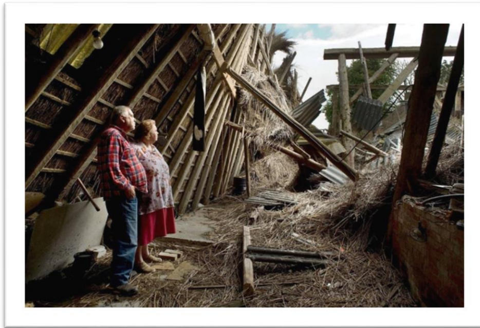
Figure 6. Tiemen and Alie Meulema is staring at their collapsed farmhouse (Ebenezer 2014)
