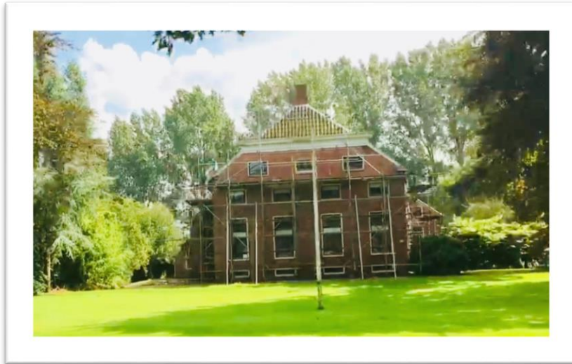
Figure 4. A big house in Slochteren with scaffoldings against it.
