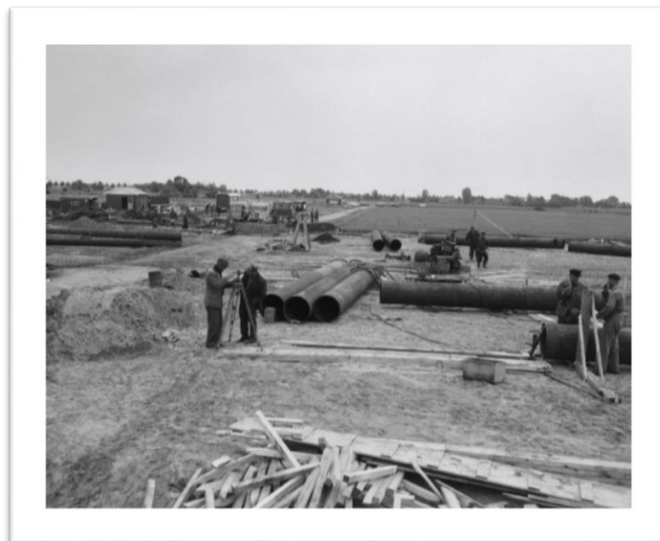
Figure 9. Setting up gas pipelines in Slochteren, Groningen in 1963 (Bilsen 1963b)
