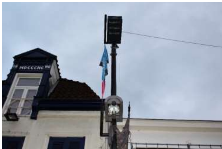
Figure 16: Sensors and smart lighting installed in Stratumseind 2.0
