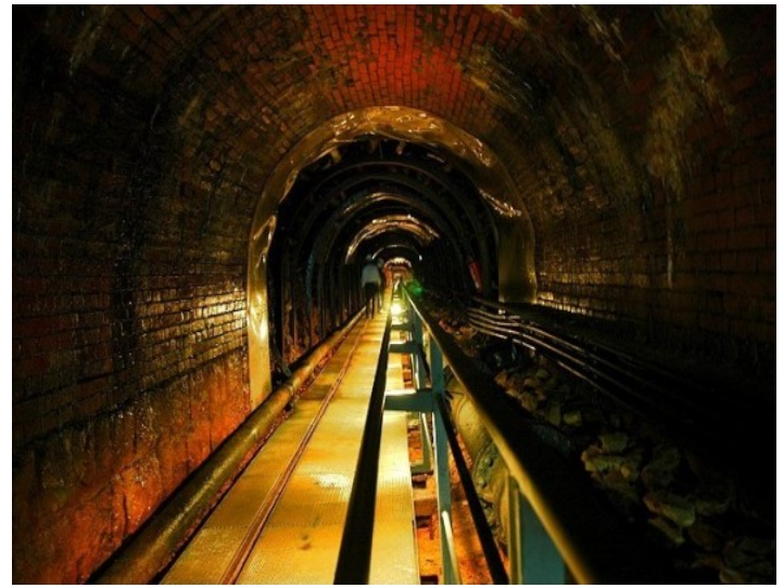
Figure 11: The 1 st mining tunnel open to the public
