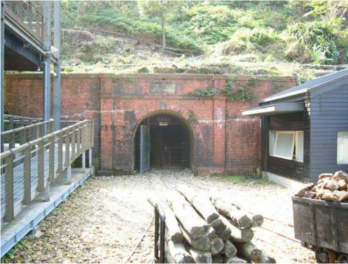
Figure 10: The BenShan Fifth Tunnel
