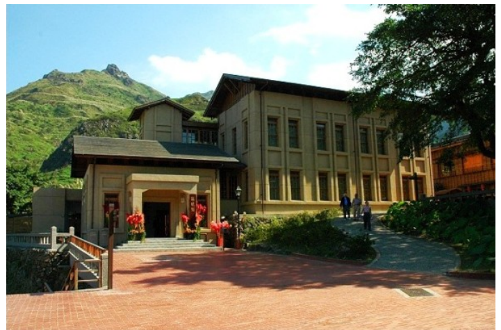
Figure 13: The Environmental Educational Centre (renovation of the old building)
