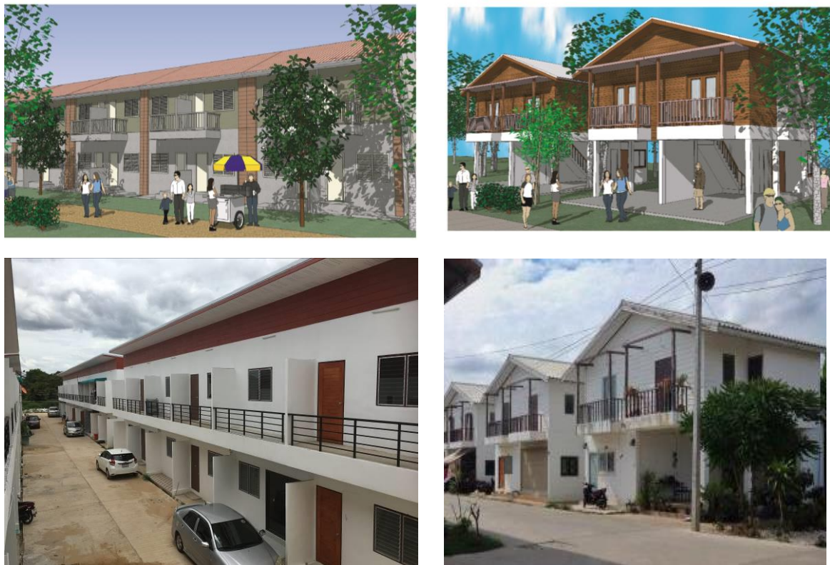
Figure 12: Render and on-site construction of Row and Twin houses Source: Render on the top CODI, 2018 – Images on the bottom the Author, 2018
