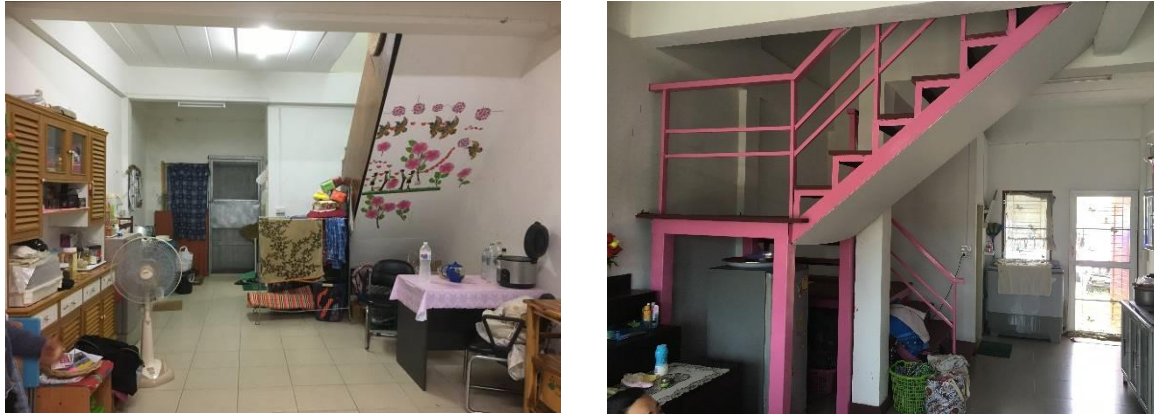
Figure 27: Comparison between the disposition of the staircase in the first and second phase Source: The Author, 2018
